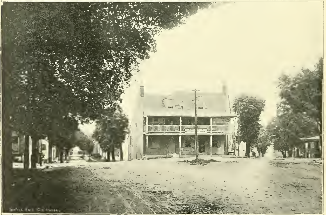
JUNCTION OF GAY STREET AND HANNUM AVENUE.
